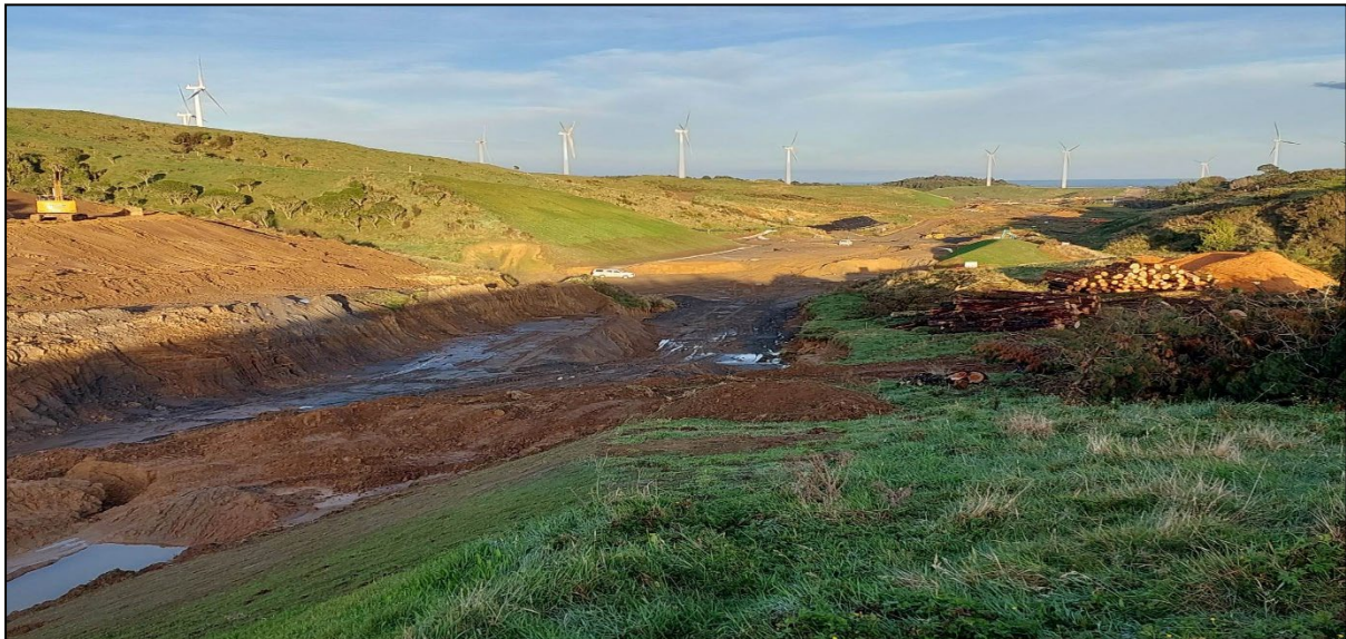
Figure 2 – Site works on Te Ahu a Turanga
